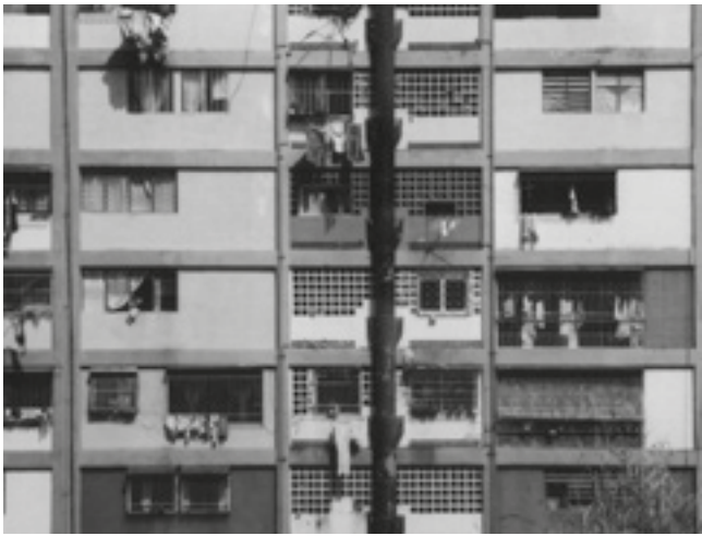
FIG. 3. FACADE MODIFICATIONS . © PHOTO: BITTER/WEBER.
