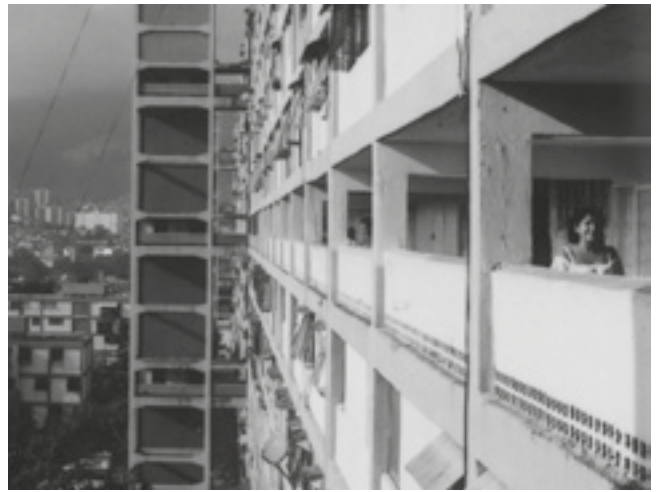
FIG. 4. WALKWAYS . © PHOTO: BITTER/WEBER.
