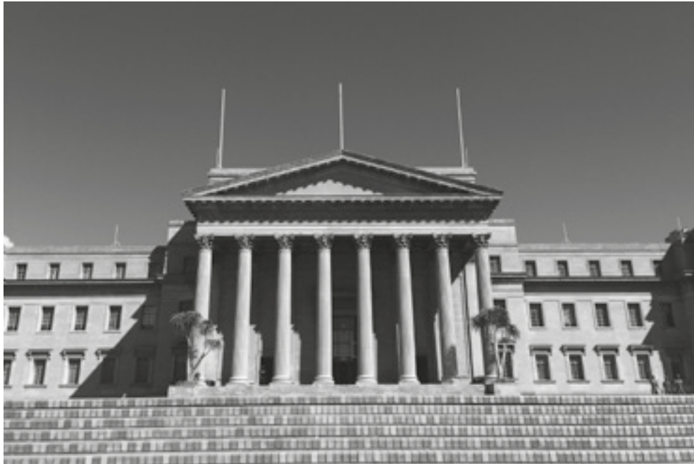
FIG. 2. NORTHERN ENTRANCE INTO THE WITS CENTRAL BLOCK. © PHOTO: NOLAN DENNIS, 2016.
